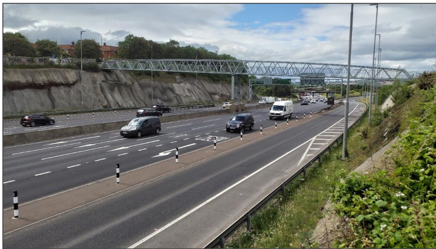
Figure 16 Shotcrete at Gateshead Quays junction
