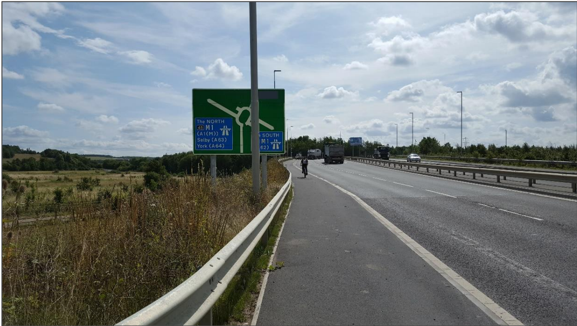
Figure 16: New footpath cycleway on eastbound approach to junction 41
