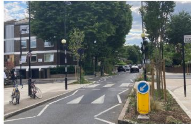
Example of raised zebra crossing with planting and cycle stands which prioritises pedestrians and encourages vehicles to slow down
