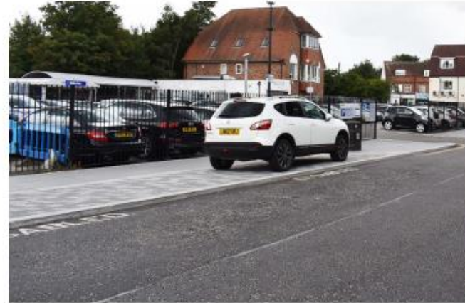
Example of inset disabled parking bays that can provide a wider footway when not in use
