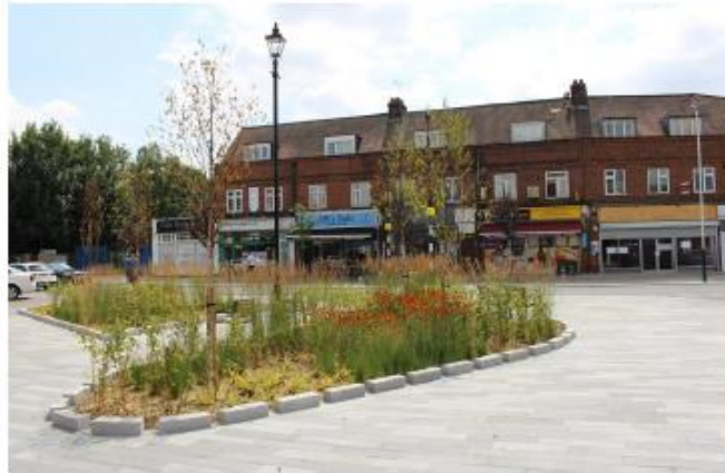
Example of rain garden to provide sustainable drainage and create a visually attractive barrier between vehicle and pedestrian areas
