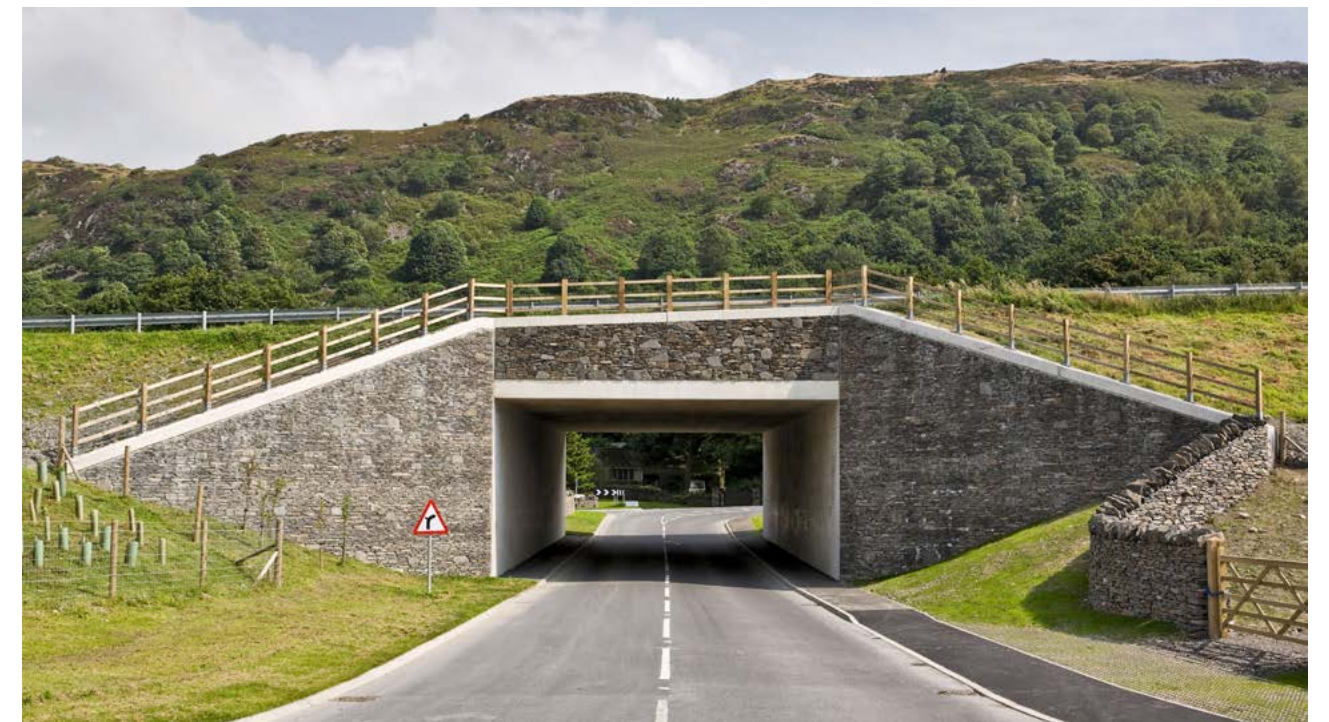
Understanding and responding to the context: Bridges on the A590 in the Lake District National Park are clad in local stone, reinforcing characteristics that make it a special place.
