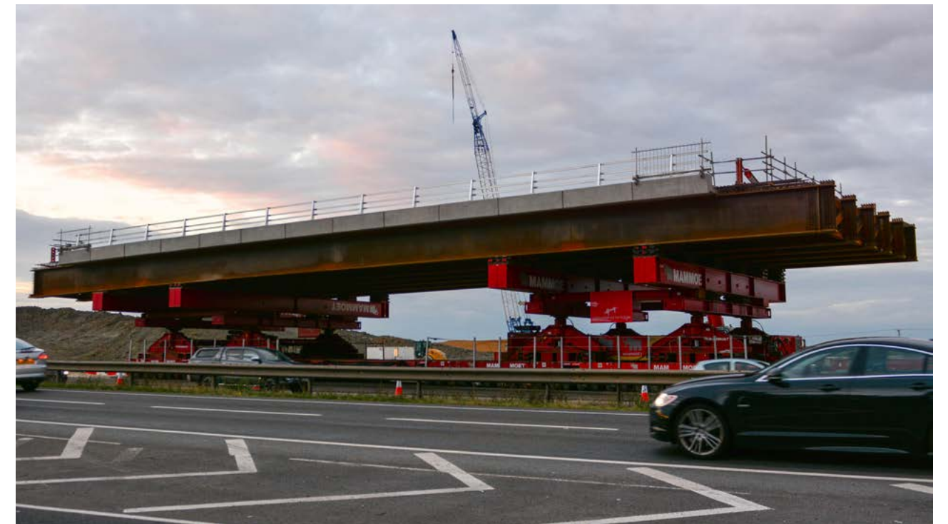
Innovation in construction: Prefabricating bridges and moving them into position over the A14 reduced the length and number of road closures required.
