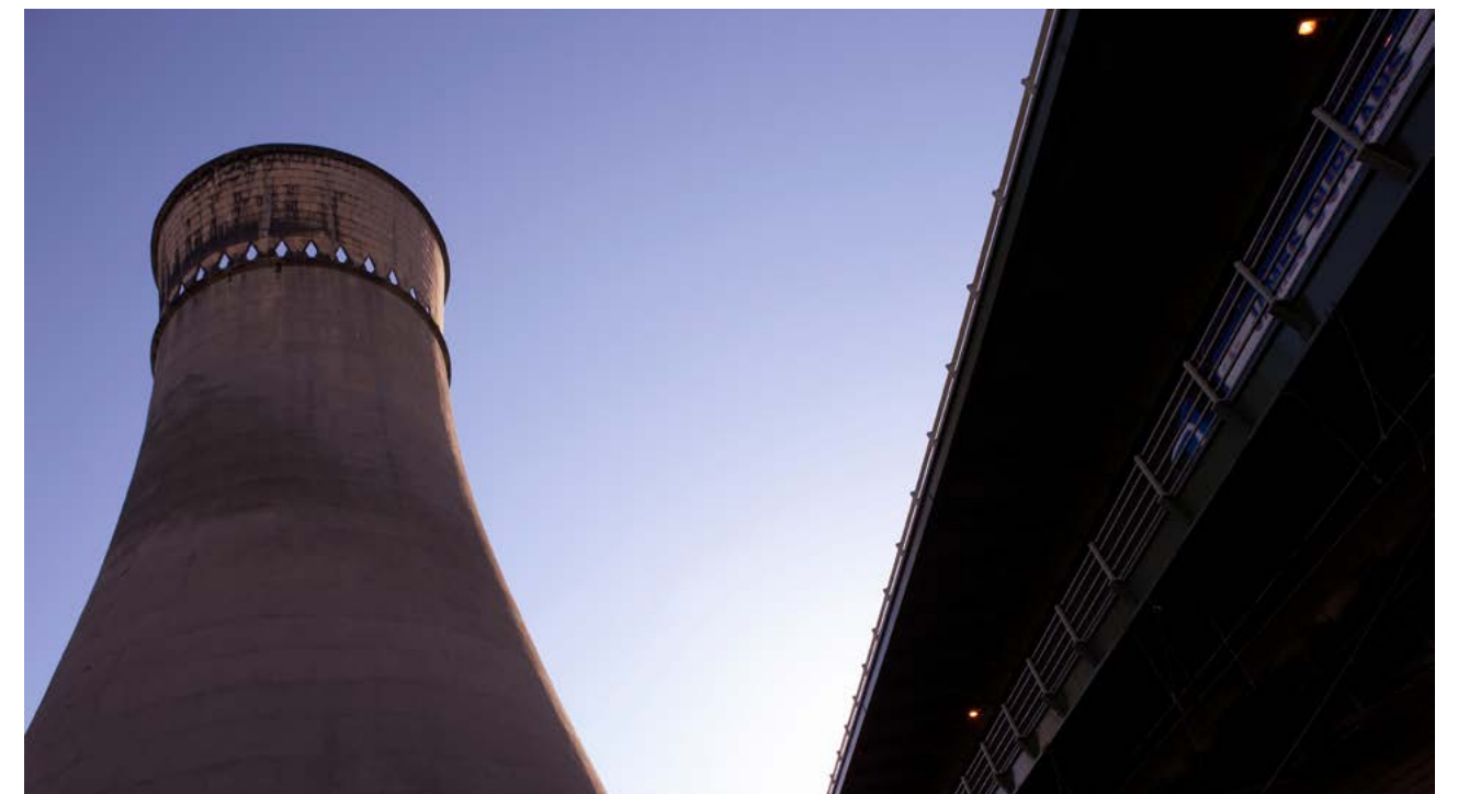
Place making: Although the adjacent cooling towers are now demolished, the M1 Tinsley Viaduct (suitably constructed from steel) remains a landmark in Sheffield.
