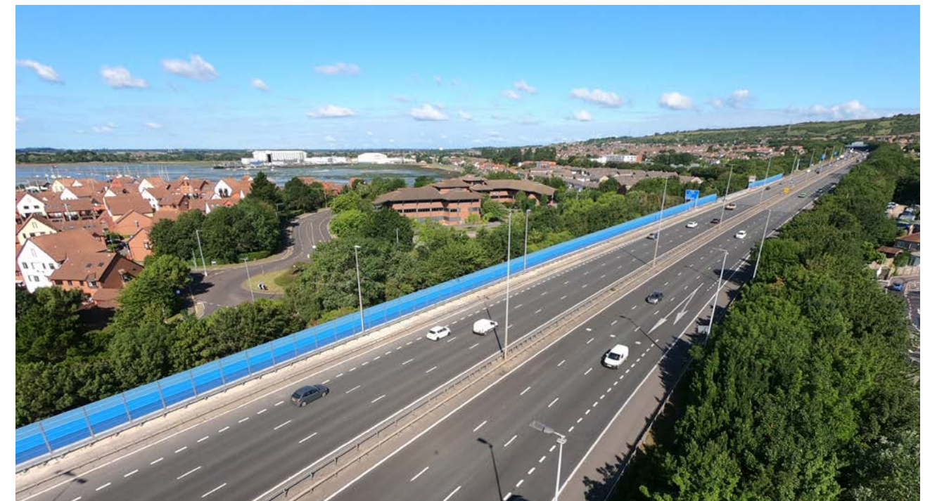
A colourful barrier to noise: The maritime themed barrier on the M27 in Portsmouth protects residents of Port Solent from noise.
