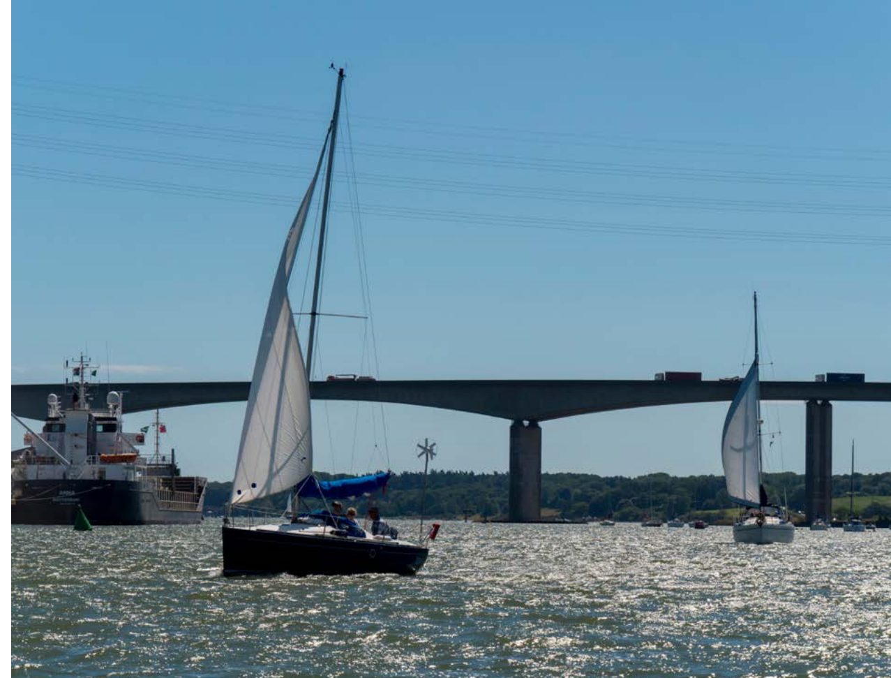
The design of the A14 Orwell Bridge, Suffolk, was reviewed by the Royal Fine Arts Commission
