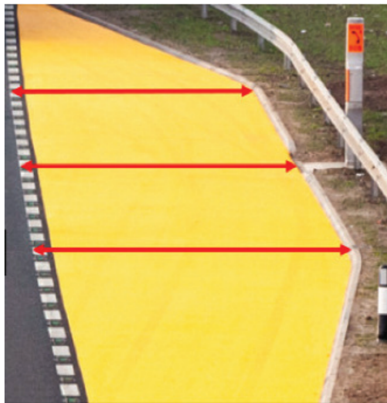
Figure 1 Emergency area width measurement locations
