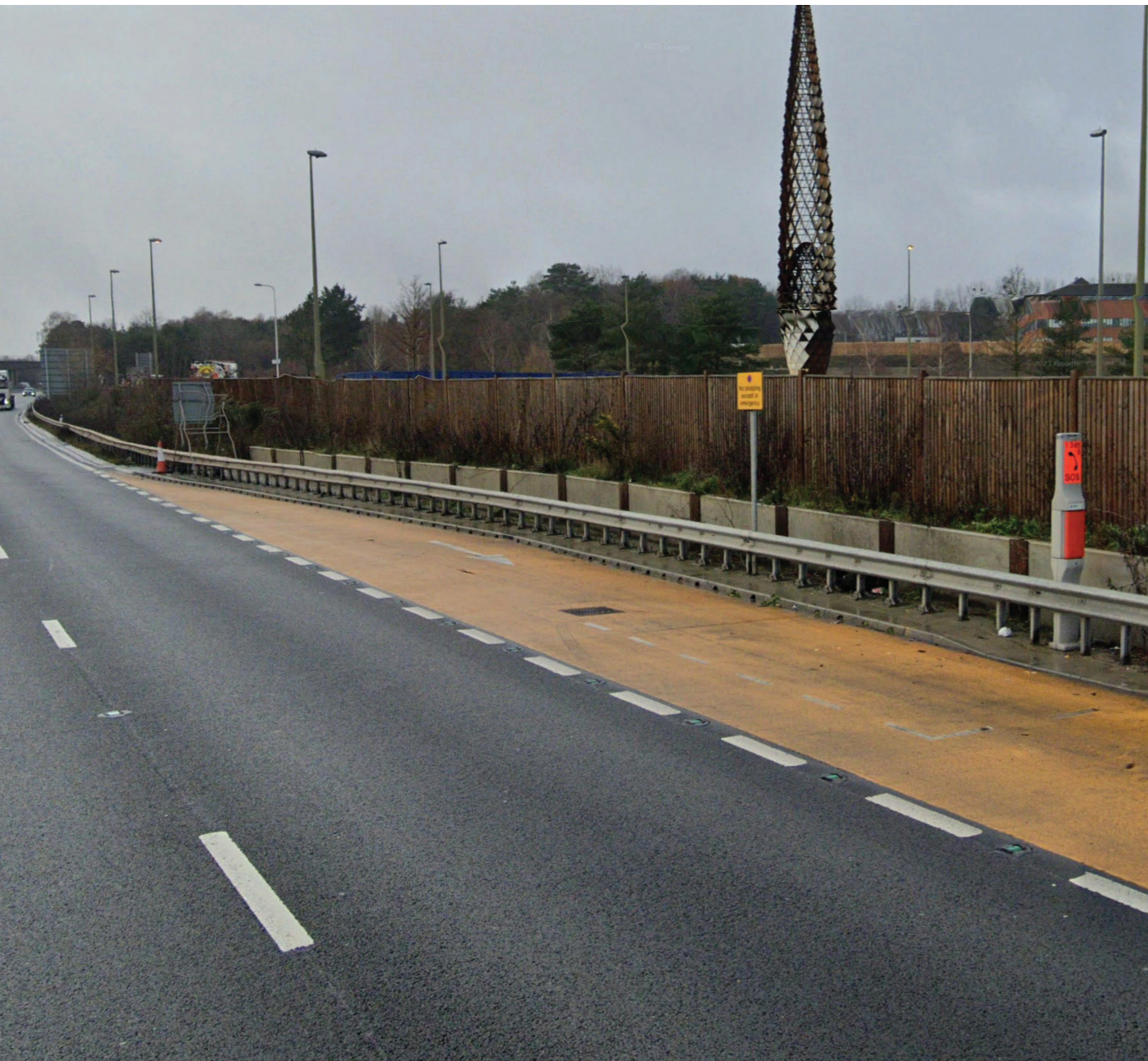
Figure 4 Emergency area M3 J3 to 2 EB B 38/5 © Google
