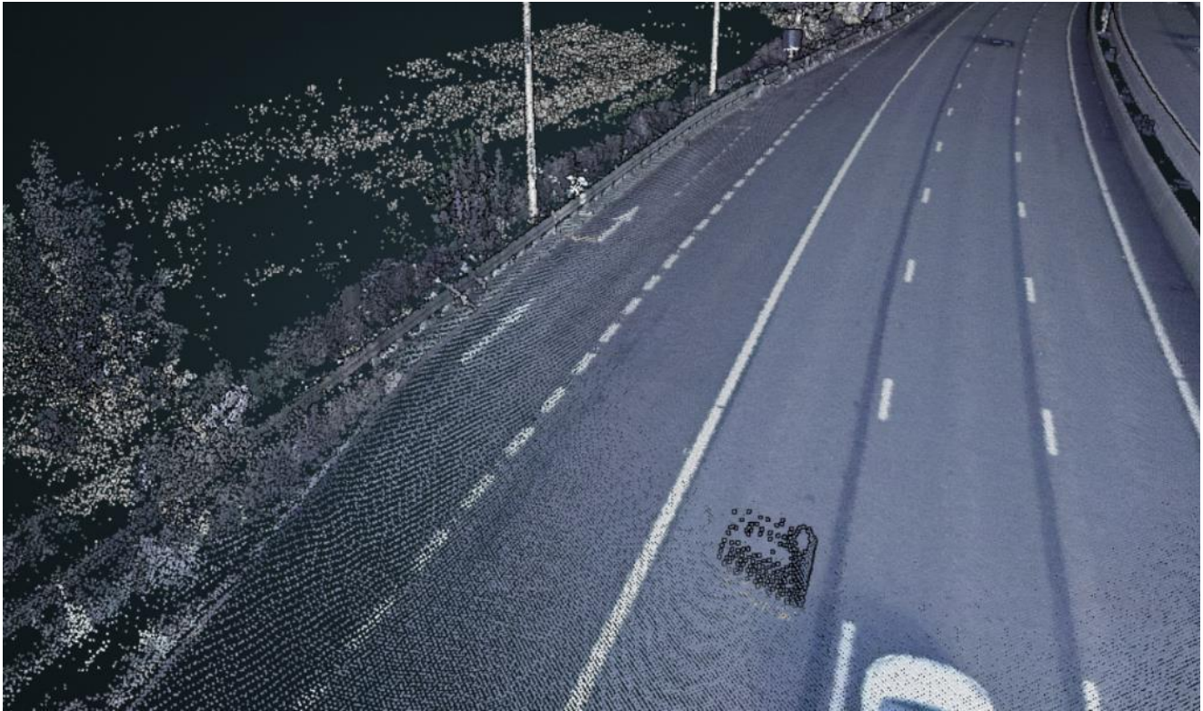
Figure 14: LiDAR image of emergency area M5 J17-J16 Northbound 133/6 B
