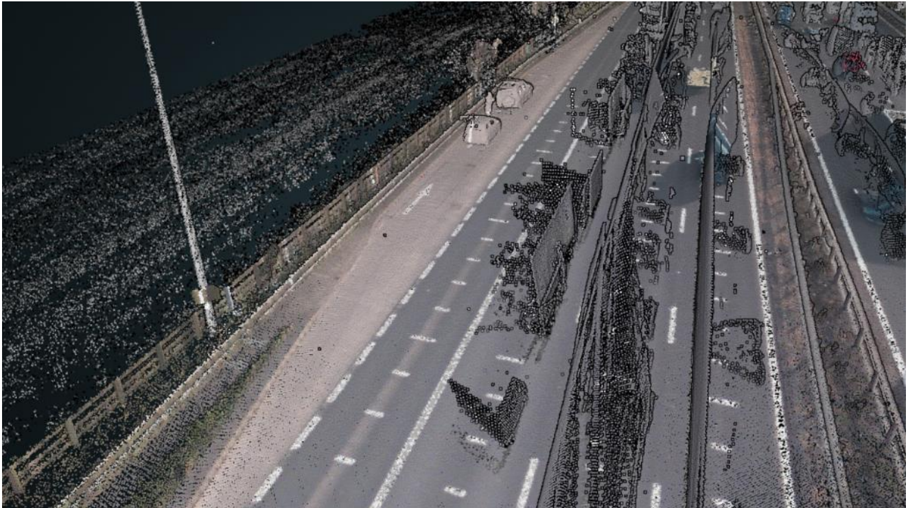
Figure 9: LiDAR image of emergency area M42 J6-J5 Southbound 28/7 B
