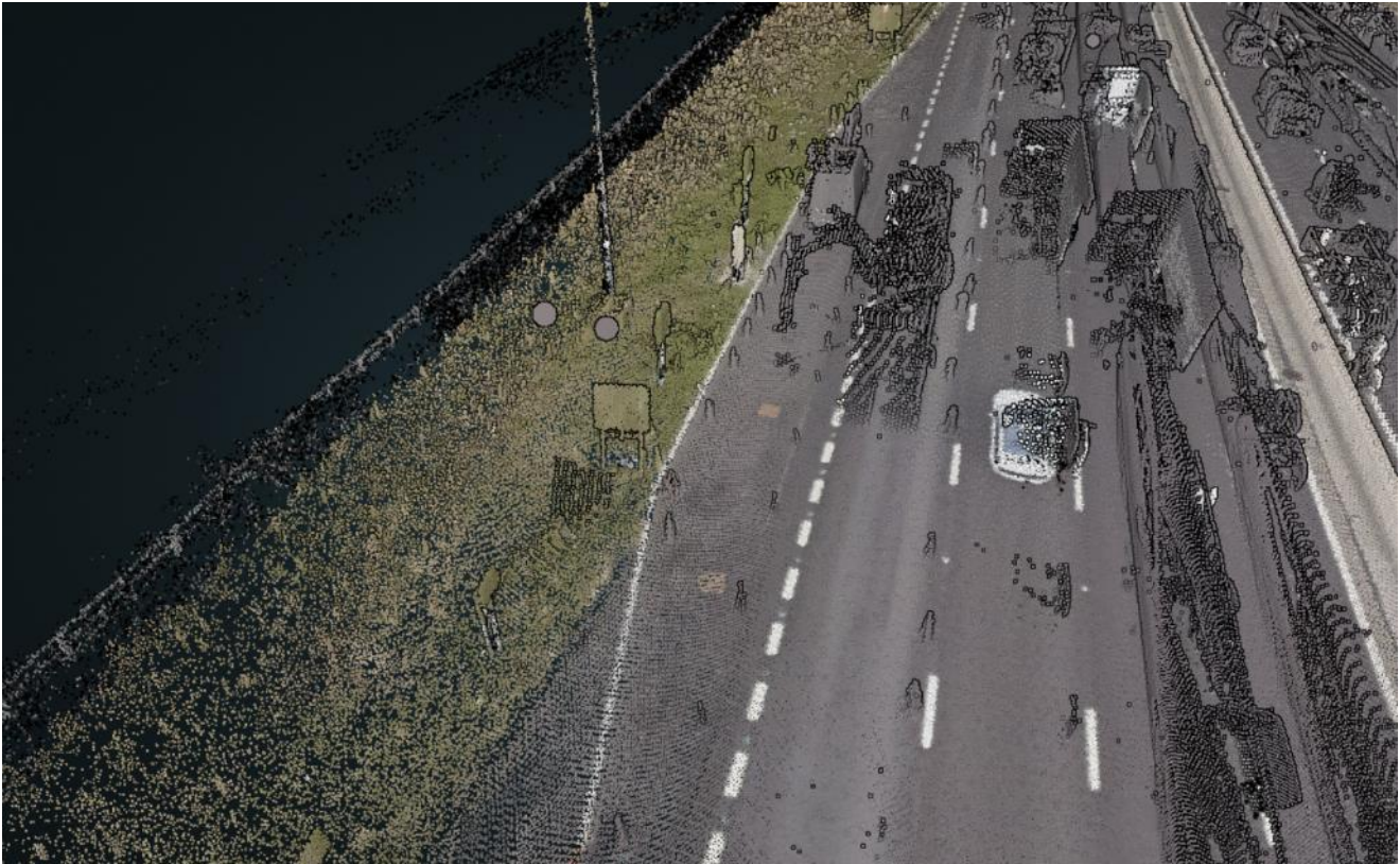
Figure 3: LiDAR image of emergency area M1 J30-J31 Northbound 241/0 A
