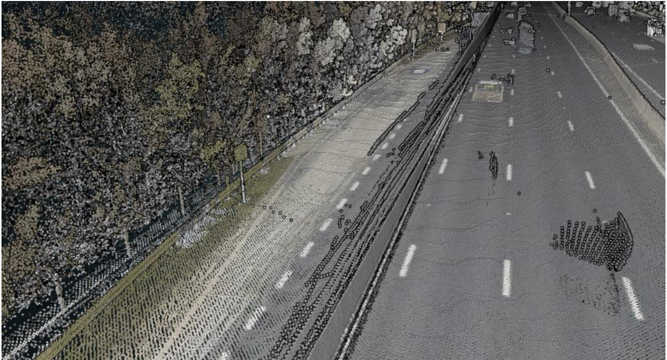
Figure 7: LiDAR image of emergency area M25 J5-J6 Clockwise 39/0 A
