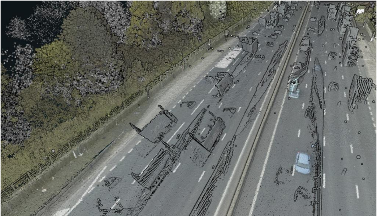
Figure 6: LiDAR image of emergency area M25 J24-J23 Anticlockwise 136/7 B
