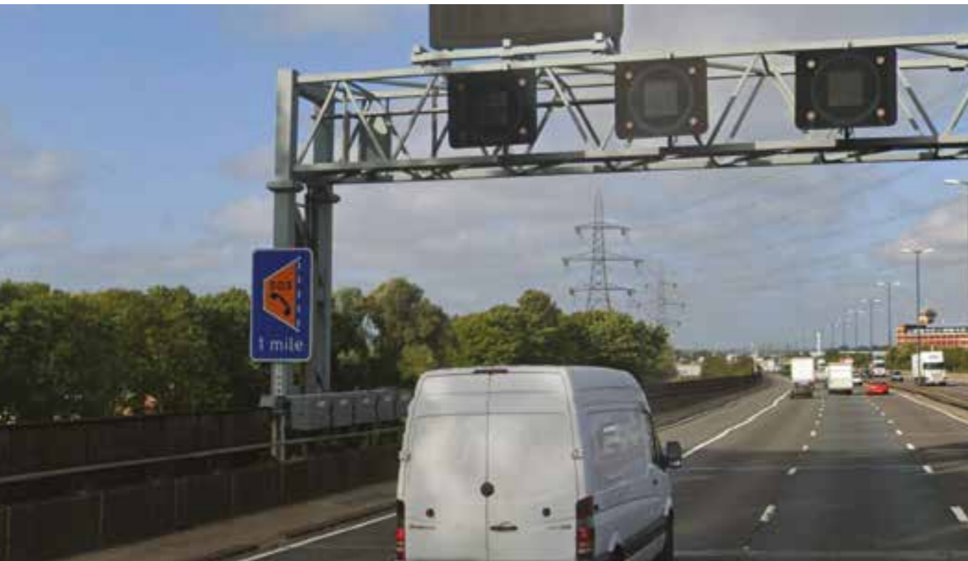
Figure 1 Emergency area approach sign on Bromford Viaduct mounted on a gantry © Google
