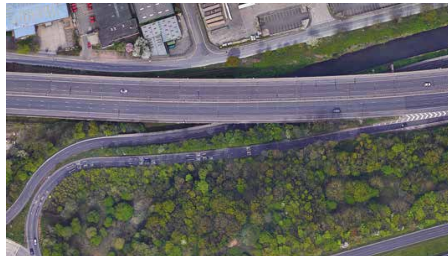
Figure 2 M6 J5 northbound exit slip road (shown on lower portion of image) an emergency area is to be implemented on this exit slip road © Google
